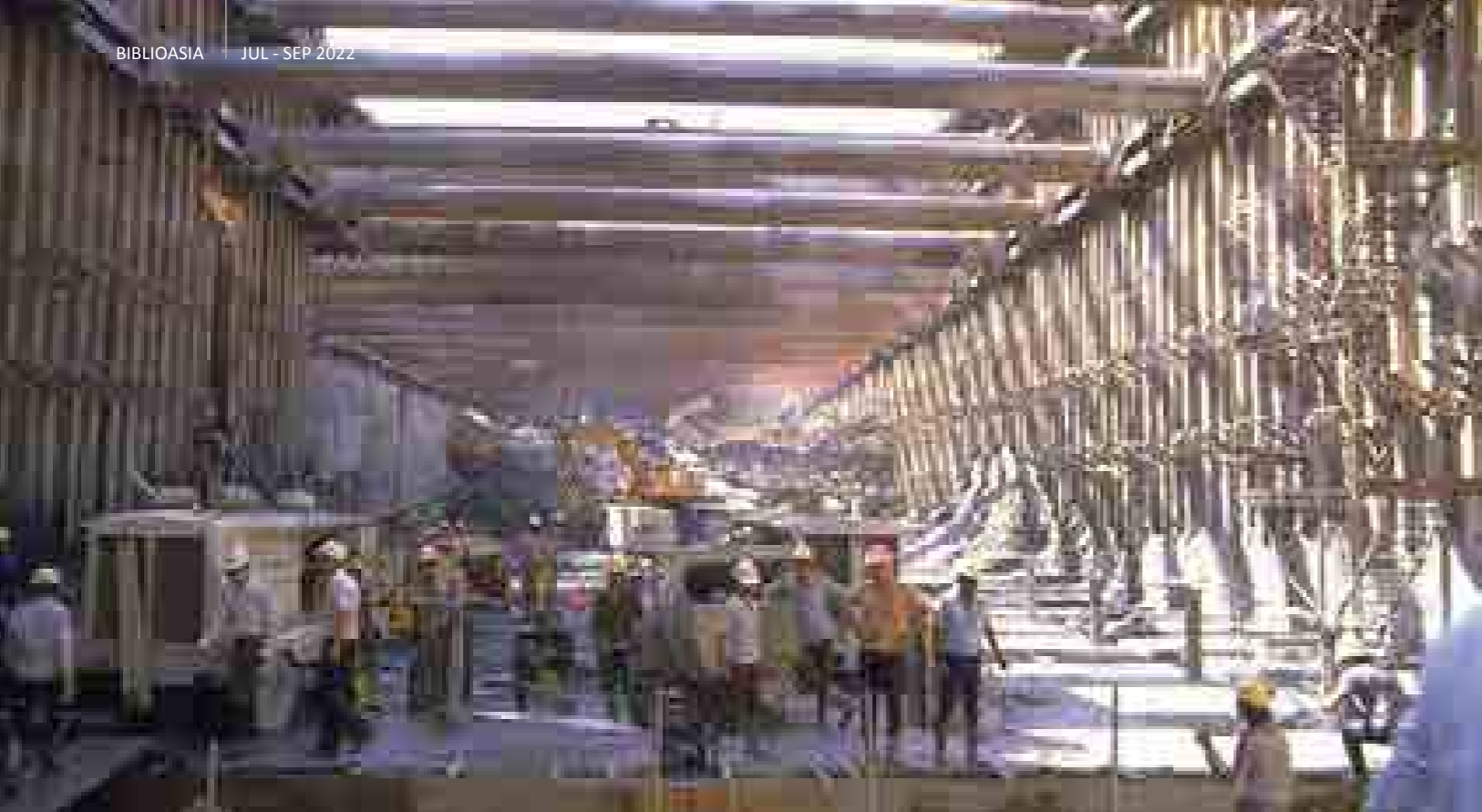
Workers constructing the underground Dhoby Ghaut MRT station, 1986. Ministry of Information and the Arts Collection, courtesy of National Archives of Singapore.
