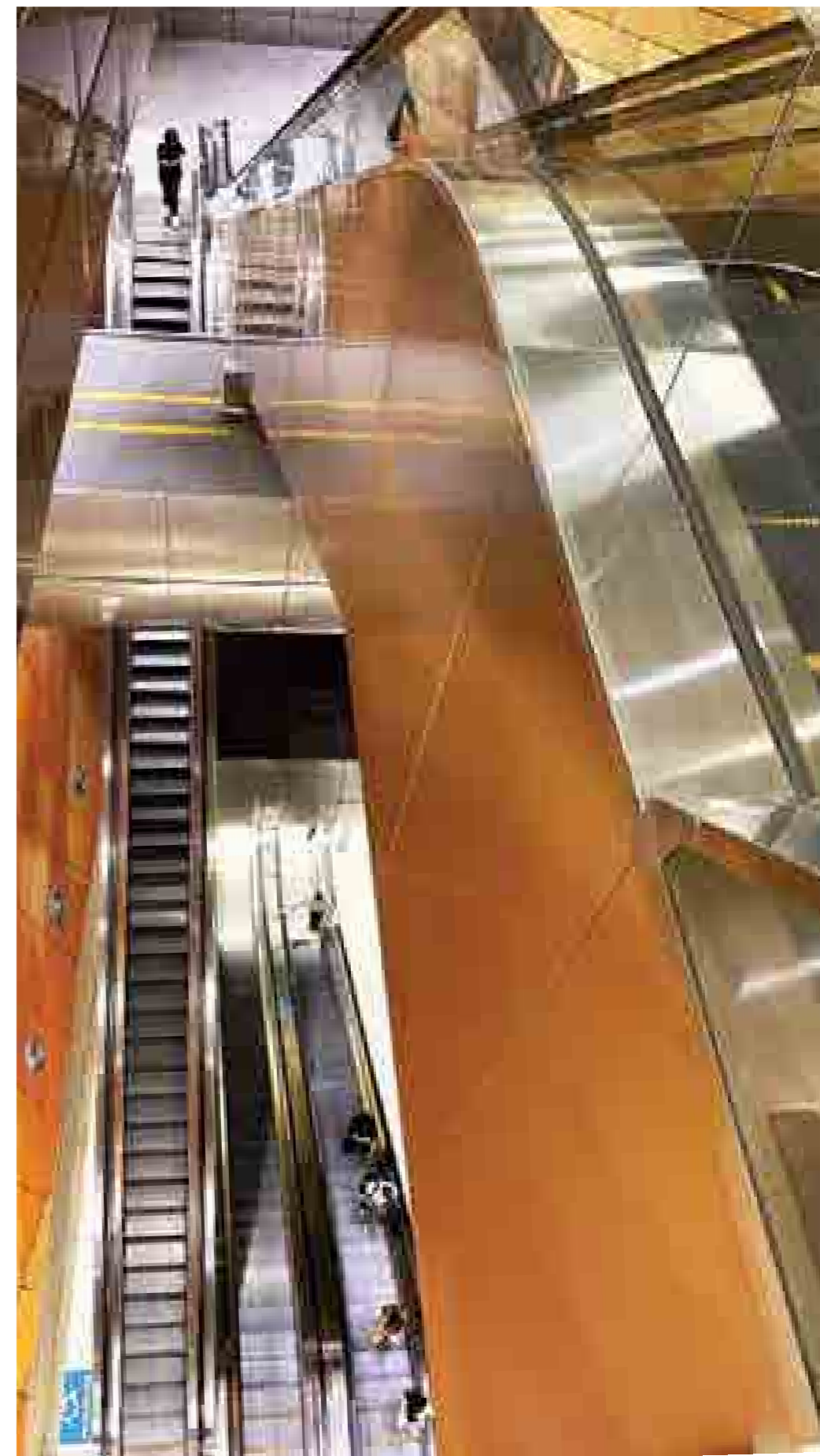
At 43 m below street level, Bencoolen MRT Station is currently Singapore’s deepest station, 2022. Photo by and courtesy of Jimmy Yap.
