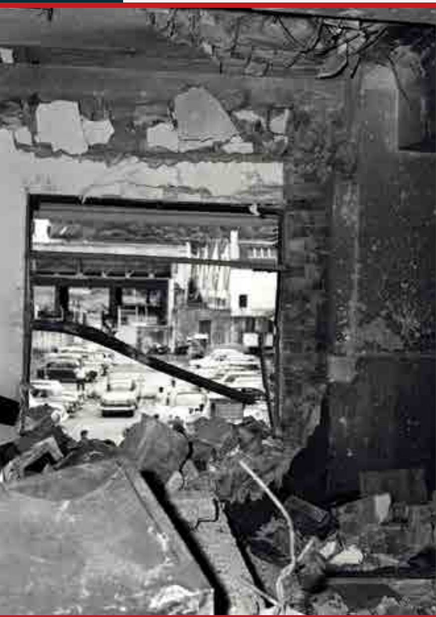
Damage from the bomb explosion at MacDonald House on 10 March 1965. The concrete wall separating the stairway and correspondence room of the Hongkong and Shanghai Bank was blown apart by the bomb, exposing the car park on the other side. Source: The Straits Times © SPH Media Limited. Reprinted with permission.
