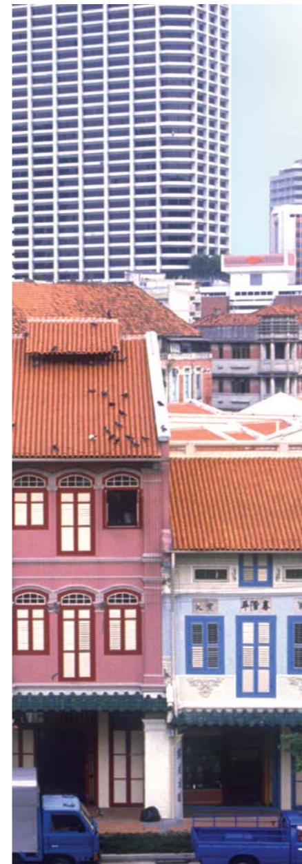
Shophouses in the Tanjong Pagar area were among the first heritage structures to be restored in 1987. MITA collection, courtesy of National Archives of Singapore.
