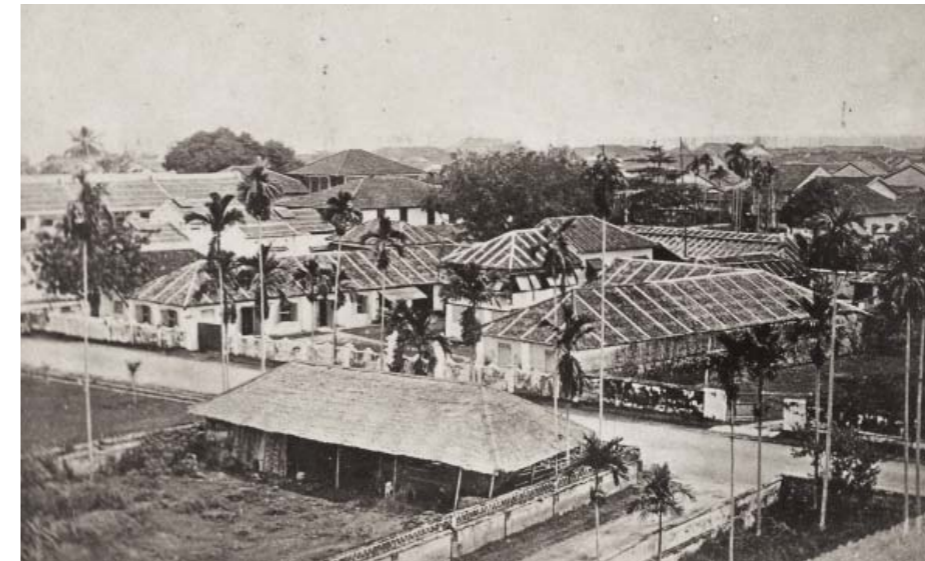
When the first Indian convicts arrived in Singapore in 1825, they were put up in convict houses located between Bras Basah and Stamford roads. Ironically, the convicts were made to build their own prison complex; work began on the Bras Basah convict jail in the 1840s and it would take some 20 years to complete. Courtesy of the National Museum of Singapore, National Heritage Board.
