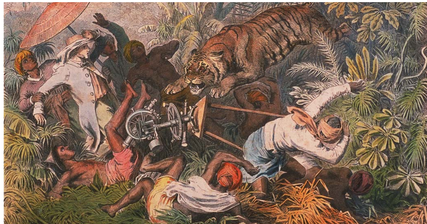
This wood engraving depicts an actual incident during which G.D. Coleman and a group of Indian convict labourers were attacked by a tiger while constructing a new road through the jungle in 1835. Fortunately, the tiger crashed into Coleman’s surveying equipment and ran away, leaving everyone unscathed. Courtesy of the National Museum of Singapore, National Heritage Board.
