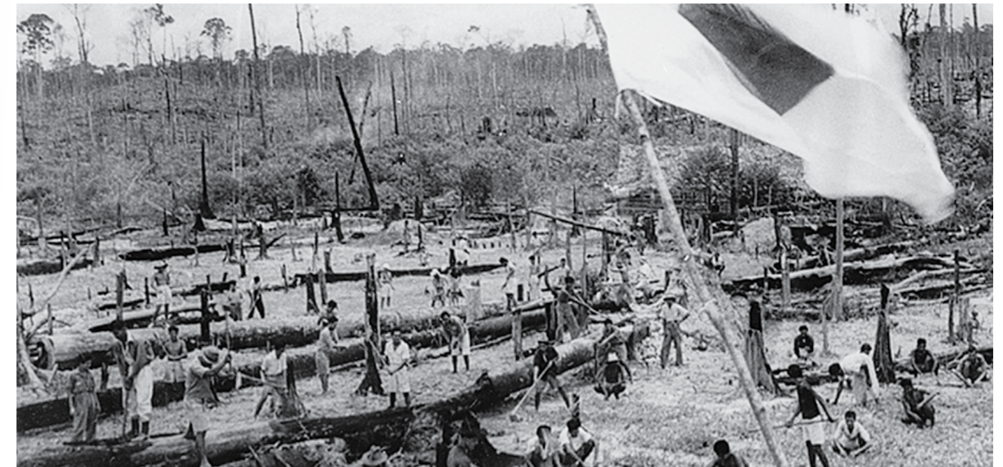
(Below) The first settlers to Bahau – mainly young, single men – had to clear the land, build a rudimentary road from the train station to the camp and set up basic infrastructure before the families started to arrive (Japanese propaganda photo). Courtesy of Father René Nicolas.
