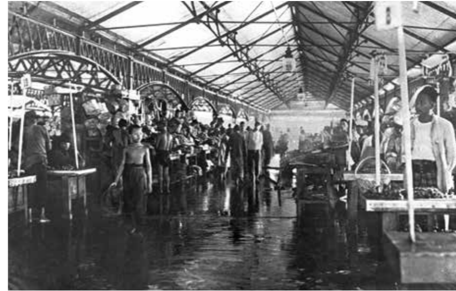
The interior of Telok Ayer Market showing the cast iron by MacFarlane and Company in Glasgow, 1910s. The market (more popularly known today as Lau Pa Sat or "Old Market" in Hokkien) opened in 1894. Courtesy of National Archives of Singapore.
