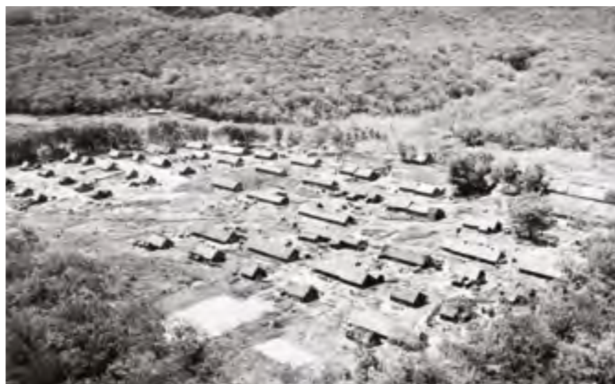
Aerial view of a newly completed village where squatters would be resettled. © Imperial War Museum (K.13796).
