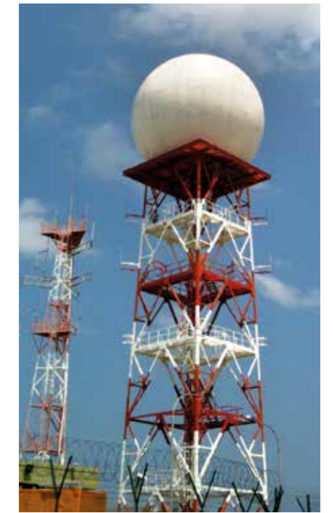
One of the most important tools used by the Meteorological Service Singapore to study the weather is the Doppler weather radar shown here, which is able to detect the motion of rain droplets, measure the intensity of precipitation and estimate wind strengths. The data allows meteorologists to monitor the development and movement of weather systems and to analyse the structure of a storm. Courtesy of the Meteorological Service Singapore.
