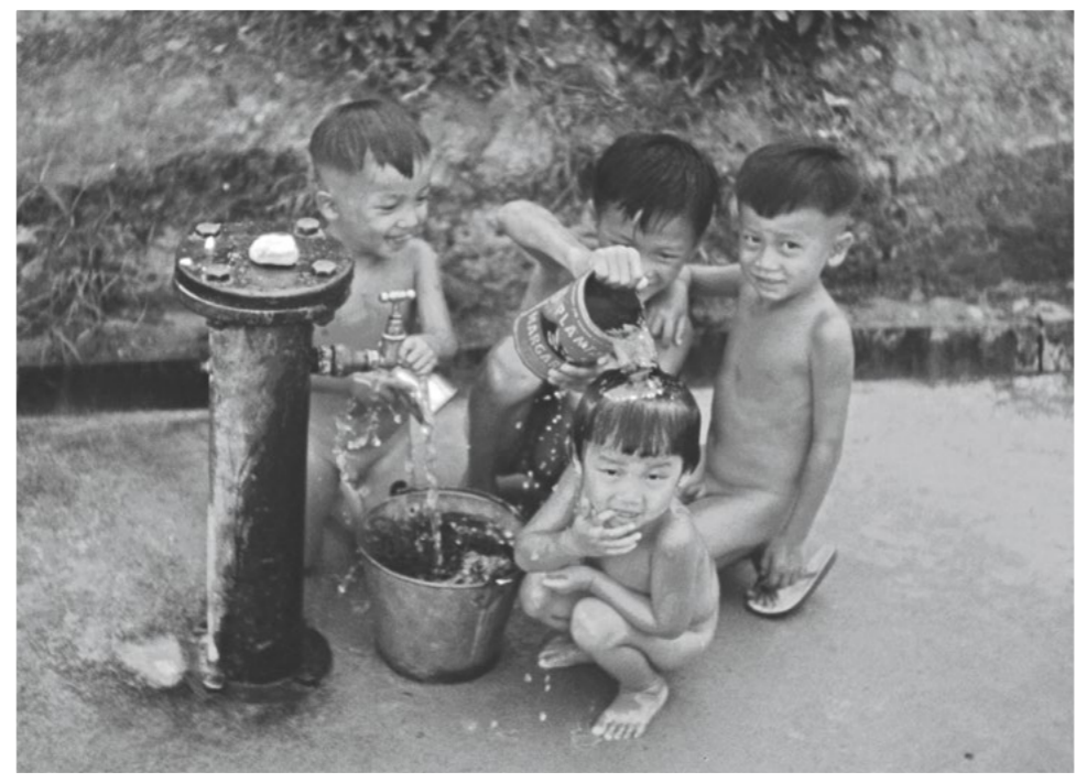
Running tap water, Seletar, 1960. The Rural and Urban Services Advisory Council had a water supply scheme in the 1960s, but some villages would not get piped water until much later. The Ralph Charles Saunders Collection, courtesy of National Archives of Singapore.
