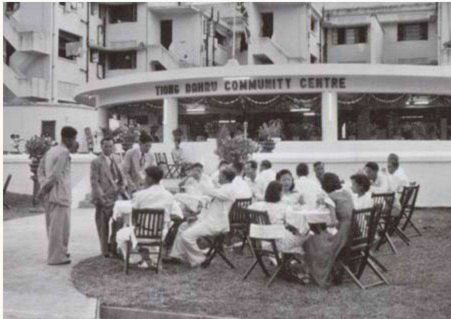
Tiong Bahru Community Centre, 1951. Source: National Archives of Singapore.
